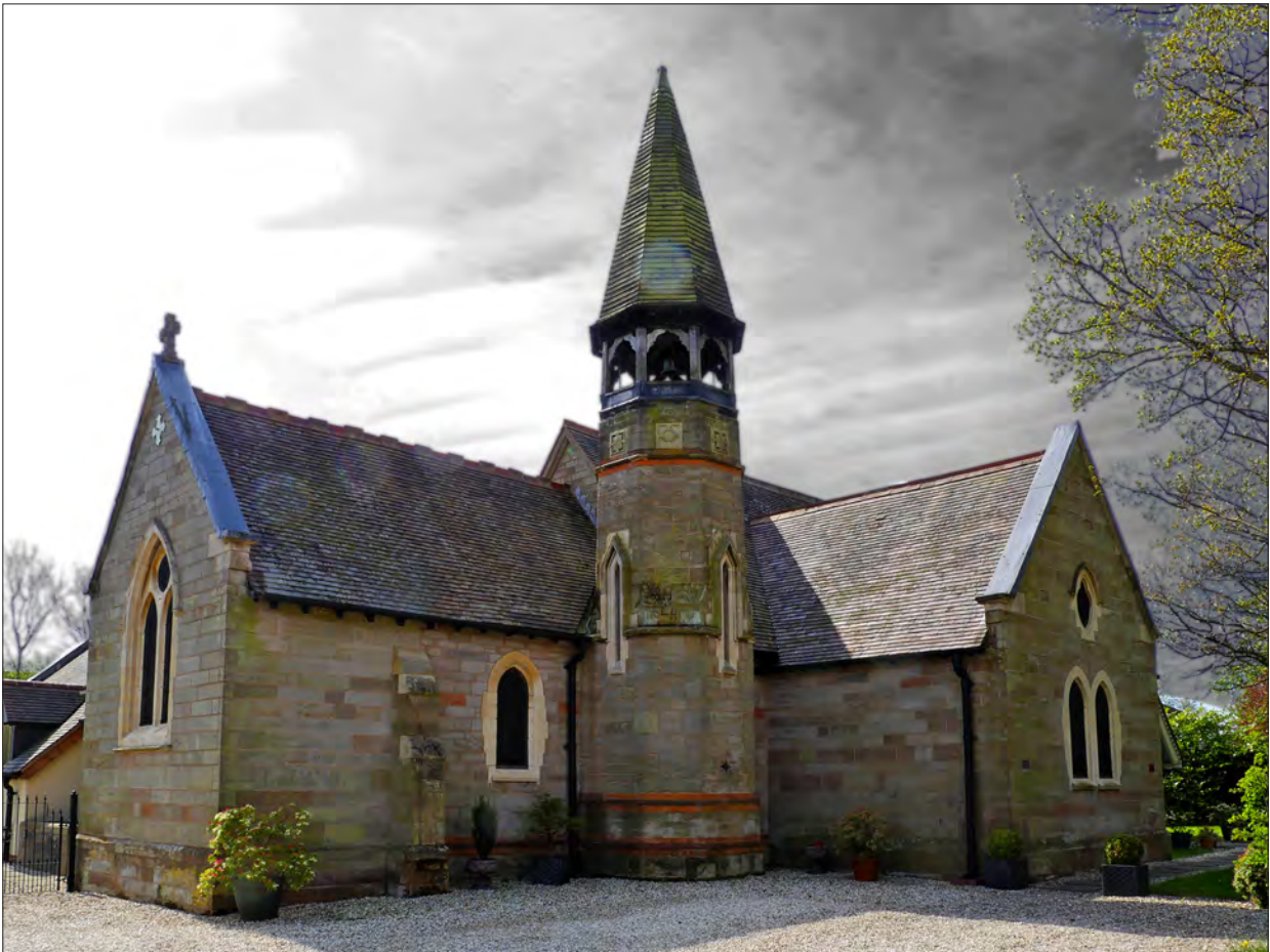
Former Blackwell church – now a live-work unit
