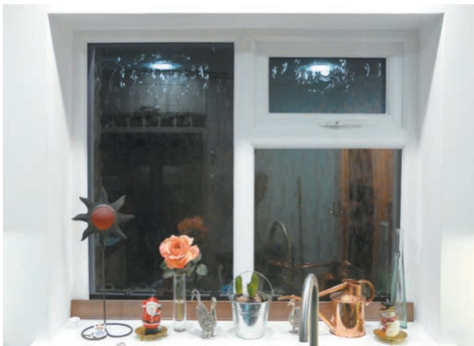
Only a small part of this window can be opened for ventilation, making it difficult for an intruder to enter.
