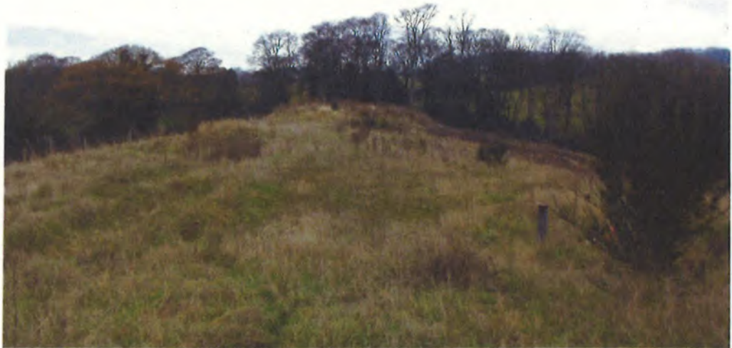
Top of embankment looking towards Right (north-west) end
