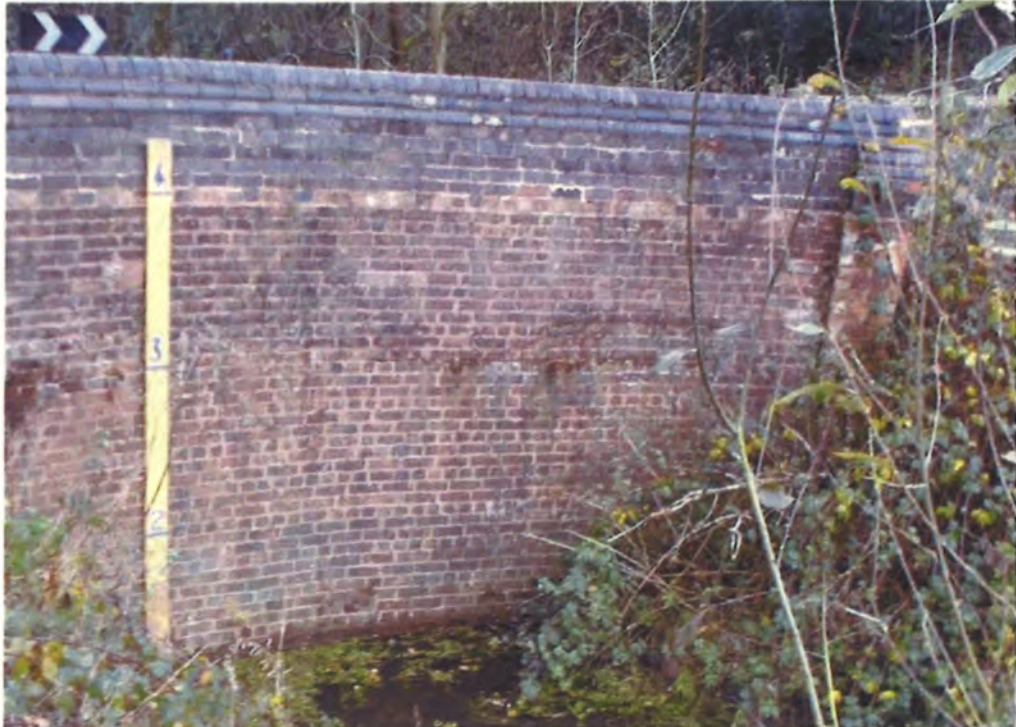
Gauge board on bridge under Alvechurch Highway
