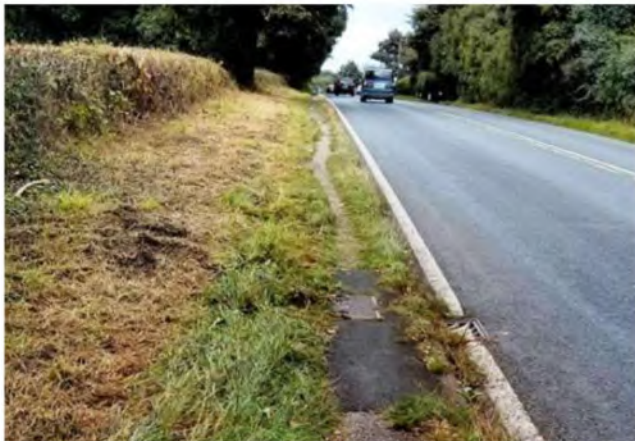
Fig 11. Public highway footpath, too narrow and too close to the main highway
