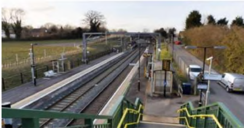
Fig 57. Alvechurch new rail station completed 2015
