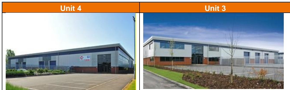
Figure 6.9 Examples of industrial units, Cofton Centre
