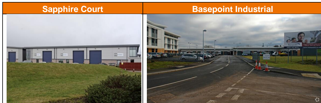
Figure 6.7 Examples of industrial units, Bromsgrove Technology Park
