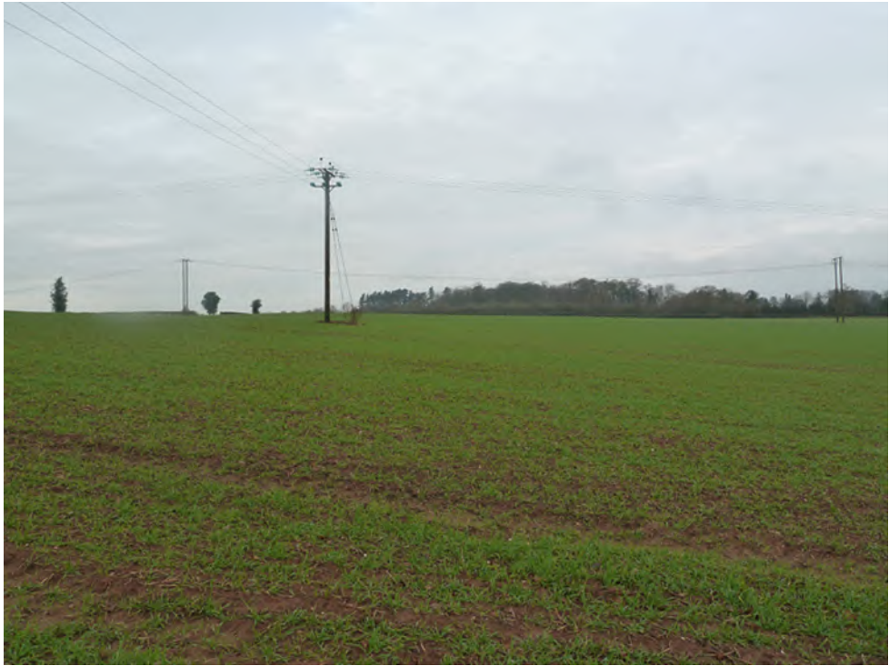
Photo WT9 View of the Water Tower from within the northern corner of the site
