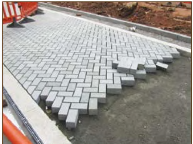
Figure 6: Resurfacing works in High Street
