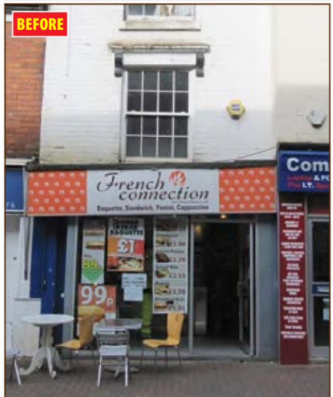
Figure 10: Improvements and new shopfront to 87 High Street
