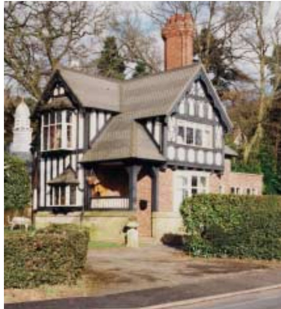
Figure 22 – Distinctive home in Shepley Road surrounded by the countryside, with hedged boundary and narrow entrance.
