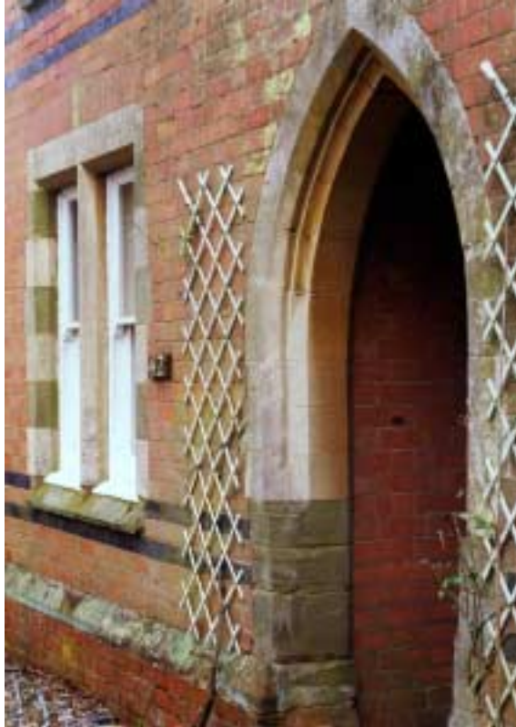
Figure 19a – Stone Mullioned Doorway, 42 Greenhill, showing there are many features that could be reflected in newer designs such as the variety of bricks used and different coloured stone.
