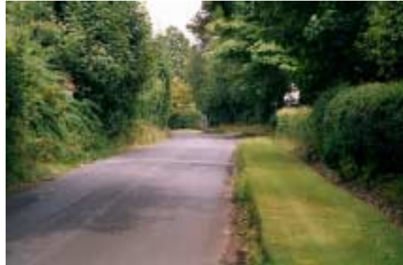
Figure 13 - Typical unkerbed road edge – to be retained and copied wherever possible. Note the bank.
