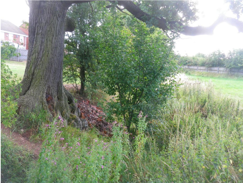
Photograph 3 - Red Ditch after first housing estate, before culvert under main road
