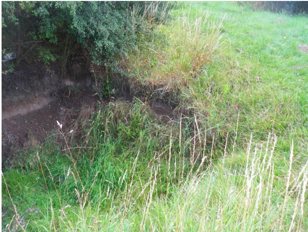
Photograph 5 - Red Ditch after first housing estate, before culvert under main road
