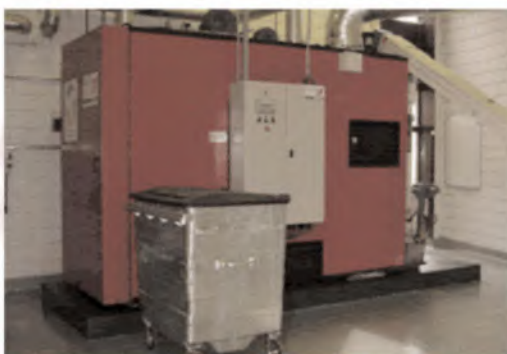
Fig. 2. At County Hall, a 700kW woodchip-fuelled boiler provides heating to the building, using locally-sourced woodfuel.
