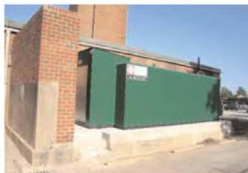
Fig. 3. A pilot project has been set up at Malvern's Chase Technology College to run a boiler on a 20% bio-diesel fuel mix.
