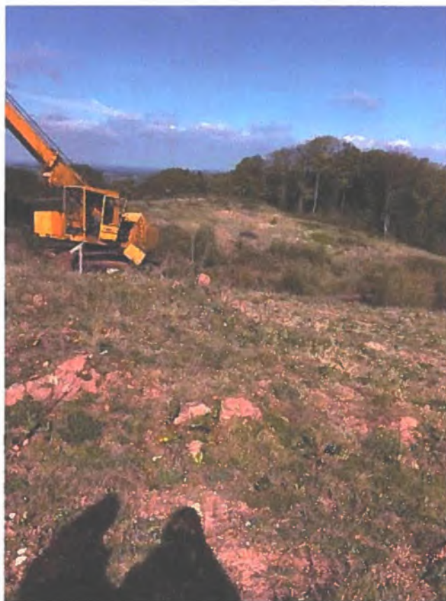
View towards dam
