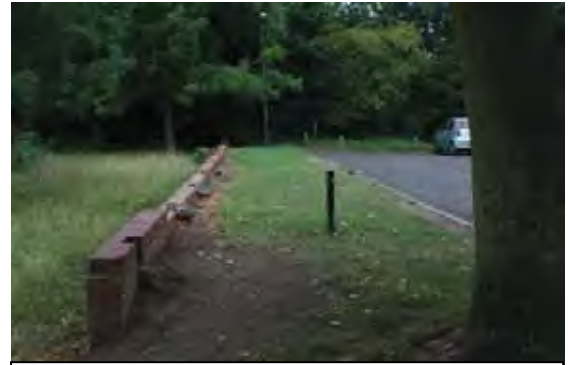
Perimeter wall along Swanslength
