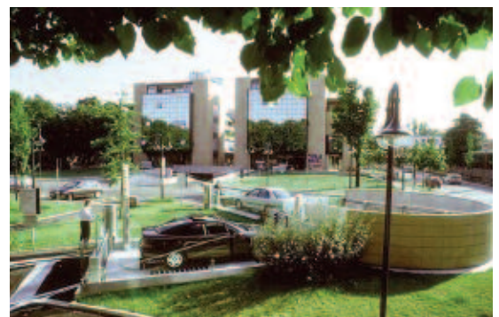
A turntable means cars access and leave in the direction of travel. It takes about 50 seconds from the request call for the car to appear.
