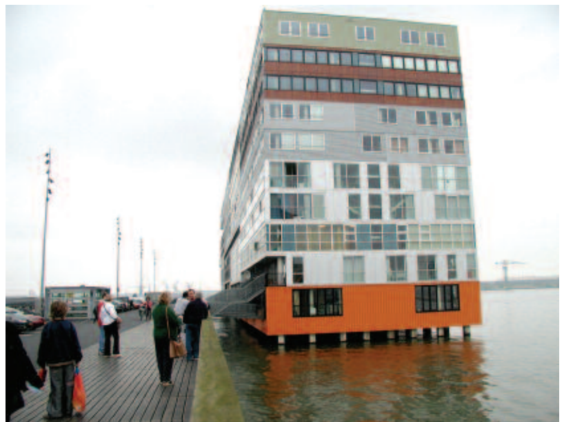
Silodam mixed-use development, Amsterdam. The entry garage to the underground car park can be seen to the left of the roadway.
