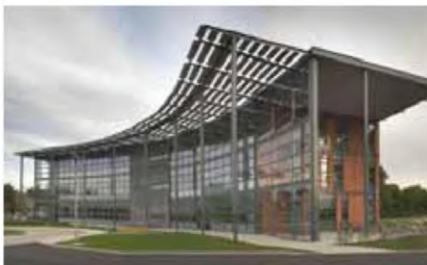
Red Kite House, Wallingford Source: Environment Agency, 2007
