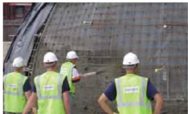
Shotcrete application Source: Shotcrete Services Ltd
