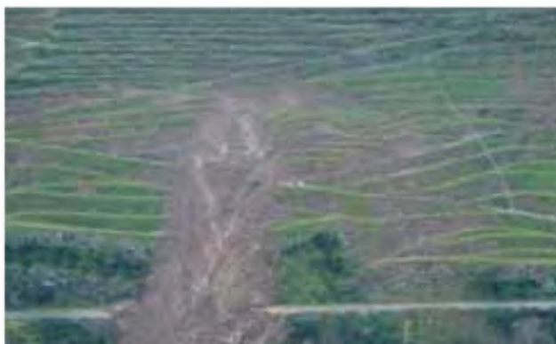
Road removed by a landslide. Villa Real district, Portugal Source: Nuno Cristelo
