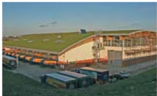
Adnams Brewery Warehouse, Suffolk Source: Lime Technology
