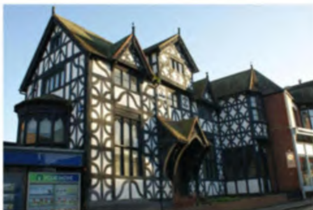
Former Hop Pole Inn, 1 New Road
