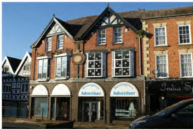
Manchester House, 3-5 High Street
