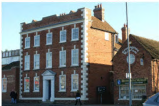
Davenal House, 28 Birmingham Road
