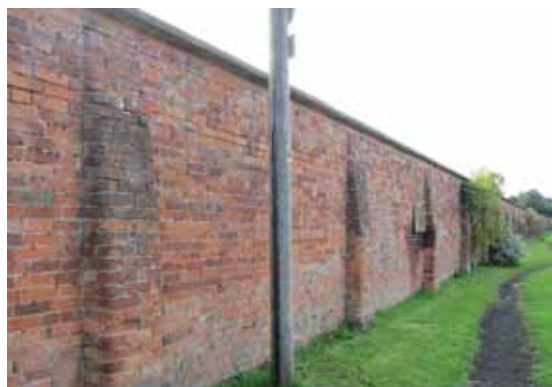
Walled kitchen garden, Holyoakes Lane
