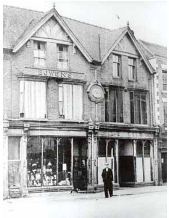
Manchester House, High Street
