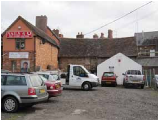
Rear of High Street
