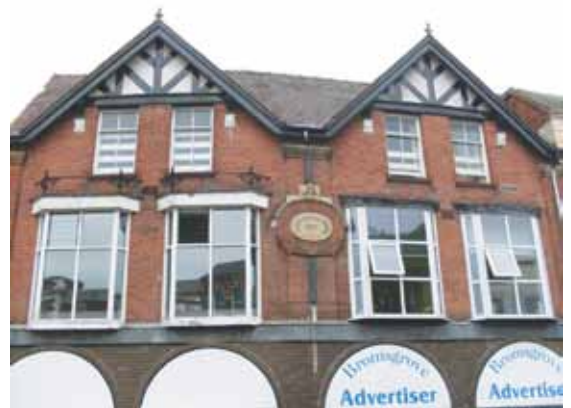
Manchester House, High Street
