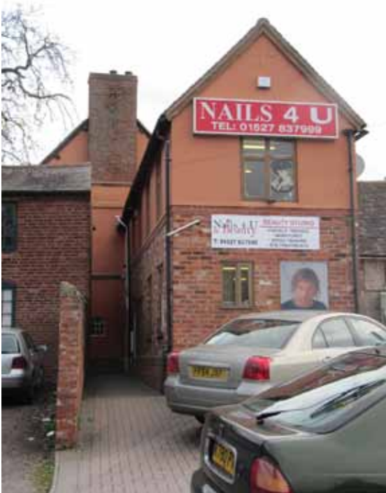
Rear of High Street
