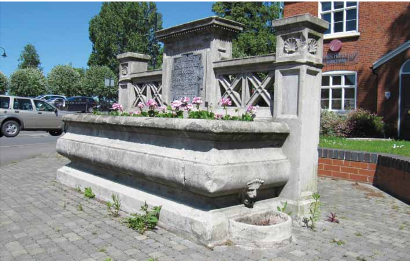
Horse Trough in front of 2 Stourbridge Road
