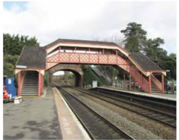
Hagley Station Footbridge
