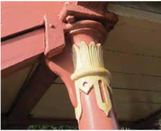
Hagley Station Footbridge
