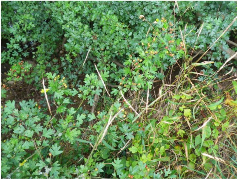
Photograph 13 - Flood defence at Paper Mill, Brooklands Lane, showing bank erosion
