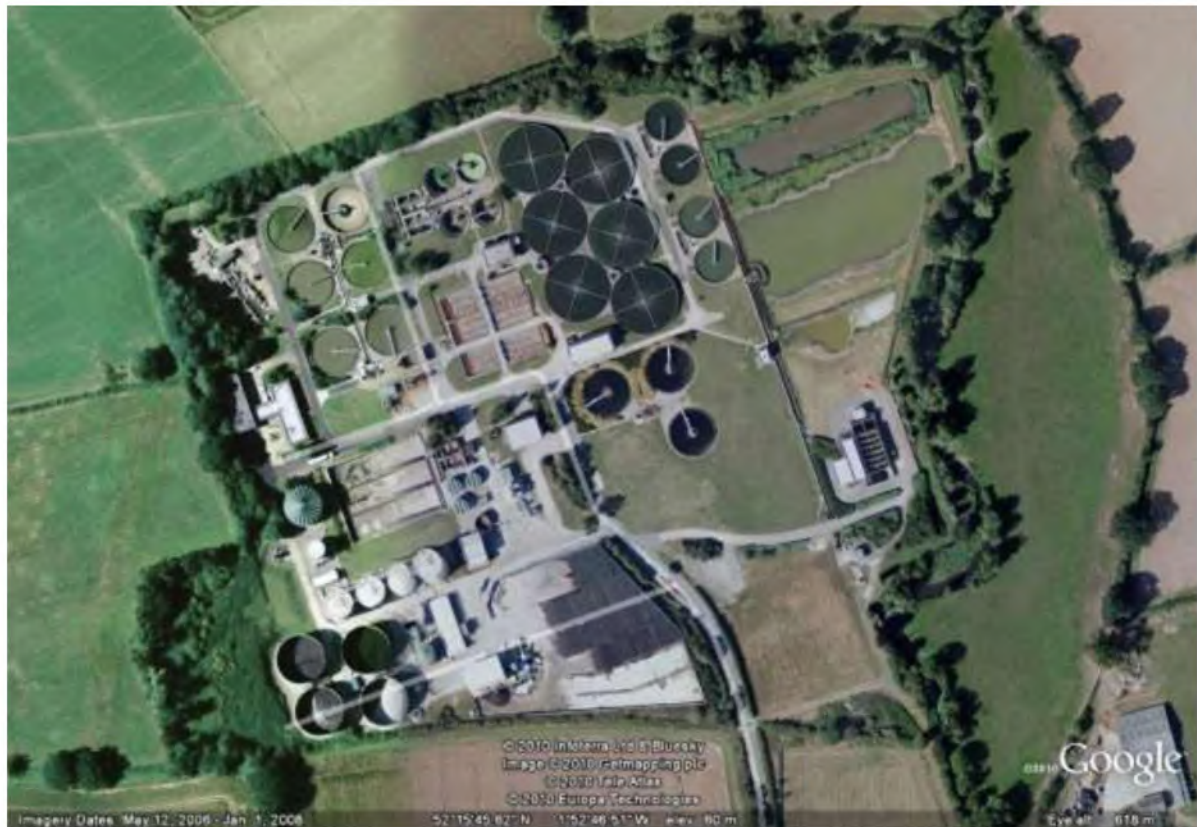
Figure 7-1 Aerial Image of Redditch (Spernal) STW
