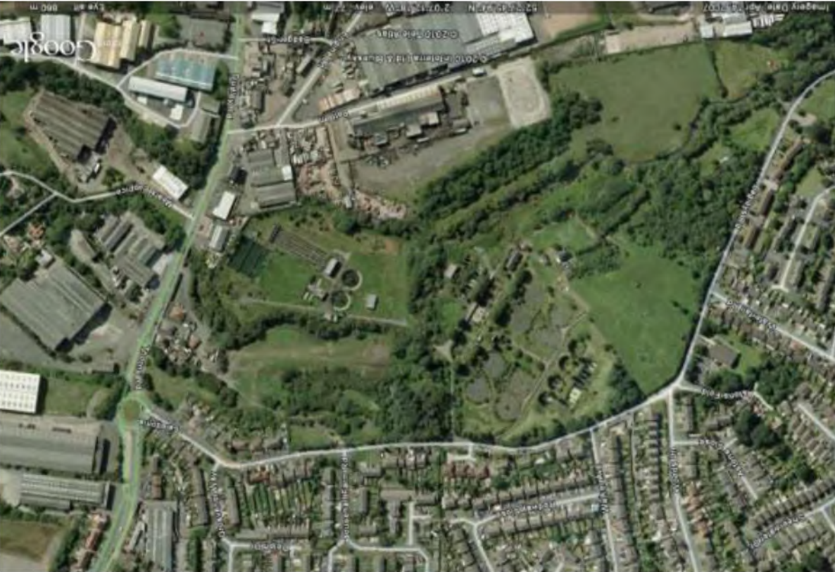
Figure 7-8 Aerial Image of Roundhill STW
