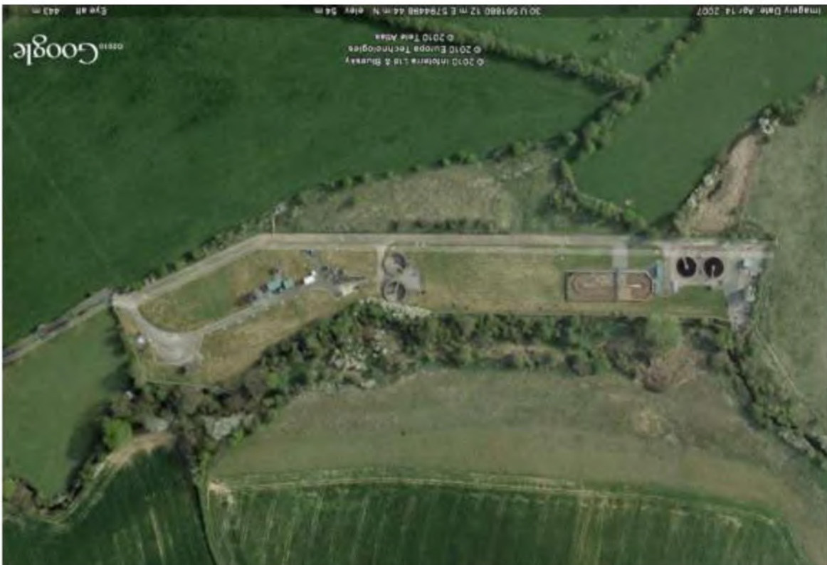
Figure 7-9 Aerial Image of Stoke Prior STW
