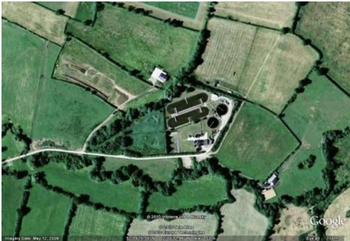
Figure 7-2 Aerial Image of Priest Bridge STW
