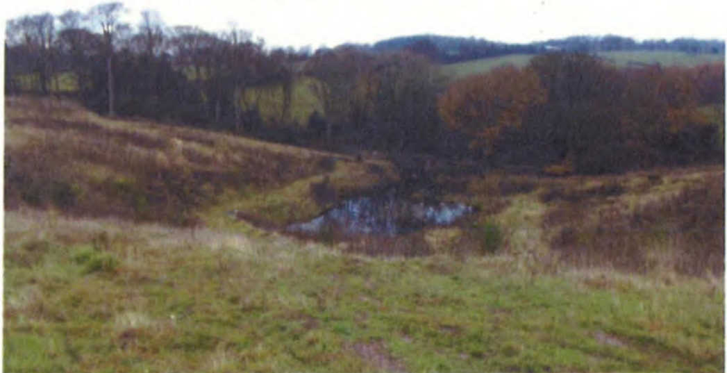
Reservoir pool area – looking north
