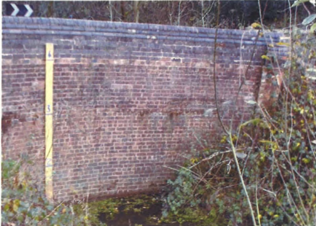
Gauge board on bridge under Alvechurch Highway
