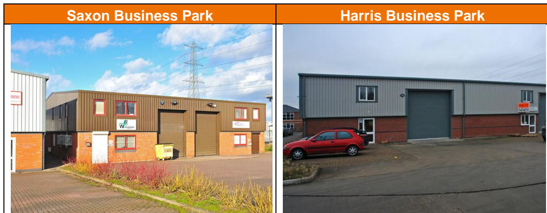
Figure 6.6 Examples of industrial units, Saxon & Harris Business Park
