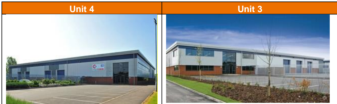
Figure 6.9 Examples of industrial units, Cofton Centre
