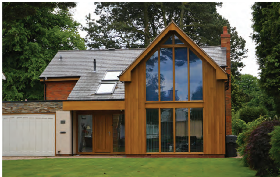
Example of a well-designed refurbishment, Old Birmingham Road
