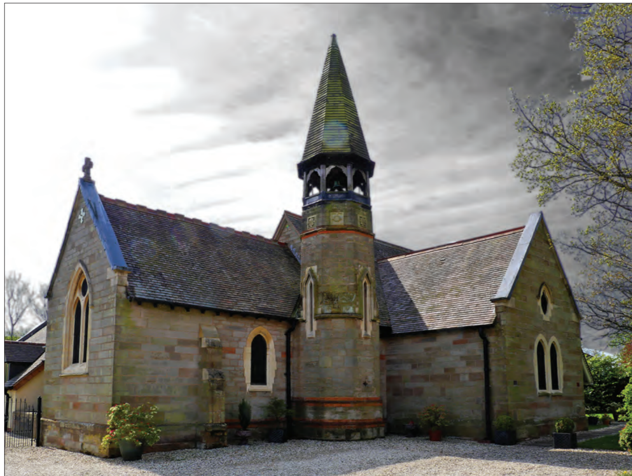
Former Blackwell church – now a live-work unit
