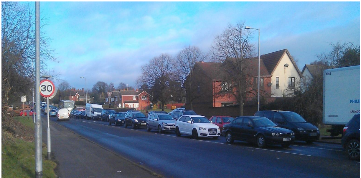
Figure 5.20 – Traffic Congestion Experienced on New Road
