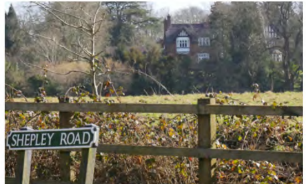
House in Barnt Green Conservation Area
