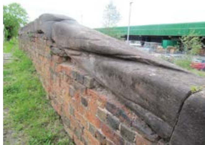
The canal arm bridge with rope marks
