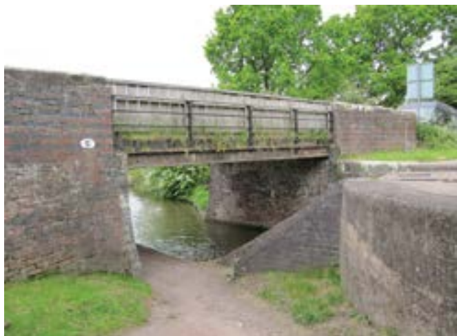
Bridge at Upper Gambolds
