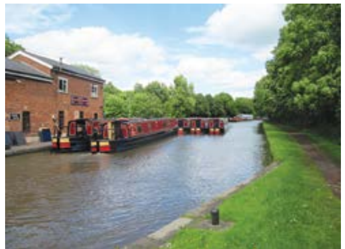
View from Bridge 44 looking eastwards along the canal
