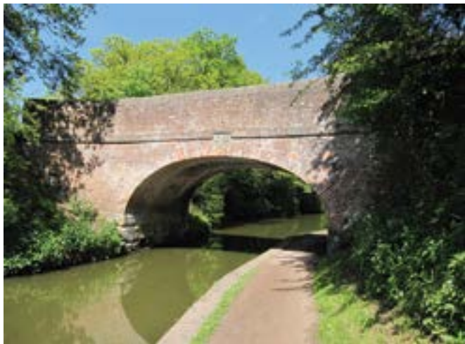
Typical Bridge, Bridge 55, with a concrete block number
