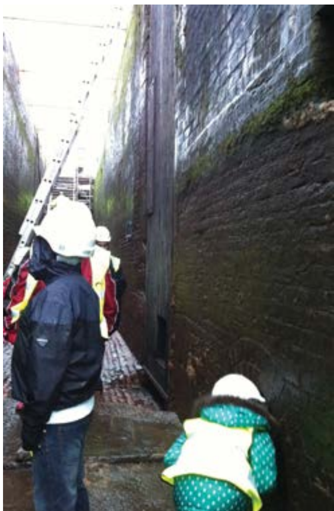
Lock 58, emptied for repairs
