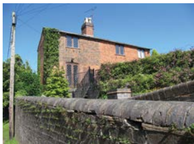
The Cottage adjacent to the Engine House
