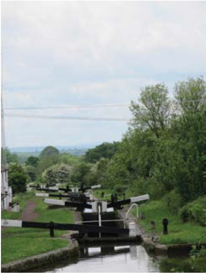
Tardebigge Flight from Bridge 51
