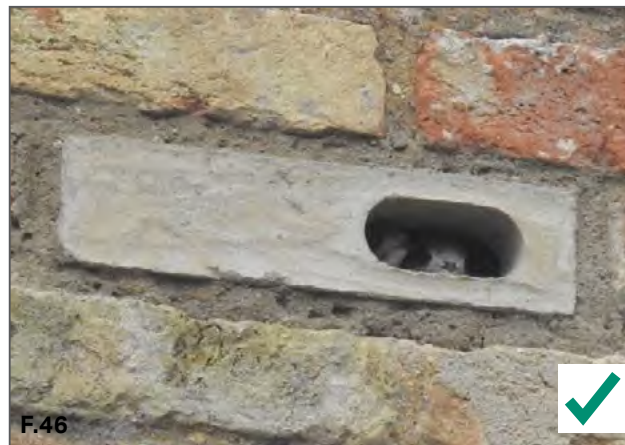
F.46 Figure 46: Swift bricks - peripheral homes (i.e. facing the open landscape) should incorporate swift bricks within their facades.
