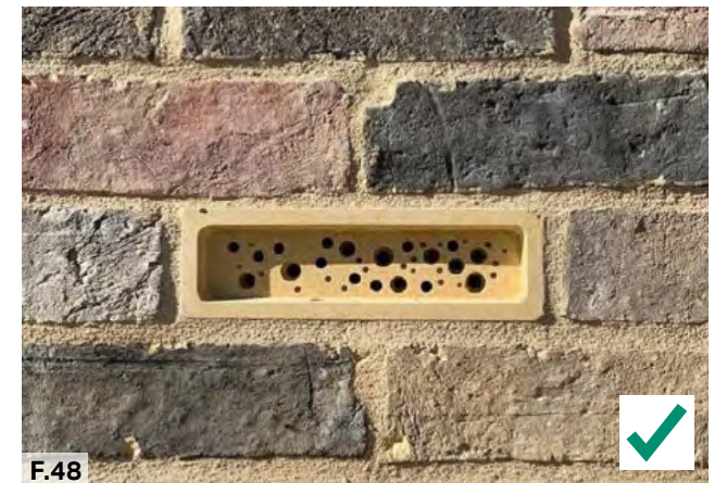
F.48 Figure 48: Bee bricks - all homes should have some form of habitat creation designed into them such as this bee brick.
