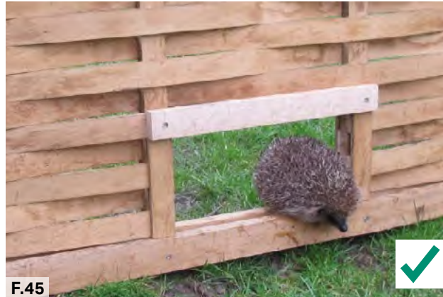
F.45 Figure 45: Fence panel with a hole at ground level to allow hedgehog movement. Multiple homes should have these to create a travel corridor for wildlife.
