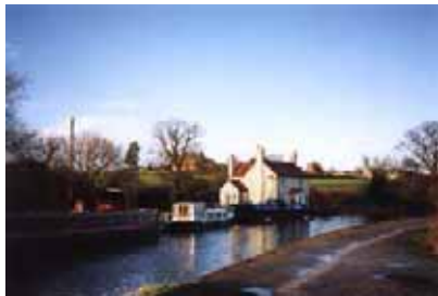
The use of the canal should be encouraged; it forms a natural boundary but is also a recreational amenity and a contributor to the commercial economy.
