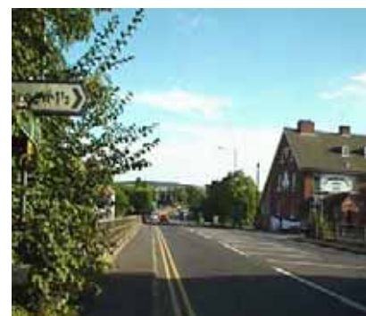
The A441 Birmingham to Redditch Road carries a large amount of traffic, connecting South Birmingham with the M42
