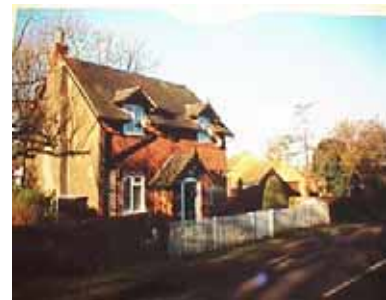
Overhanging eaves, inset dormer windows and decorative gable ends, are a local characteristic
