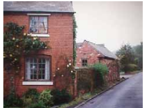
A recently-built garage, making good use of reclaimed bricks, slate roof and wooden window frames, to blend with the original cottage
