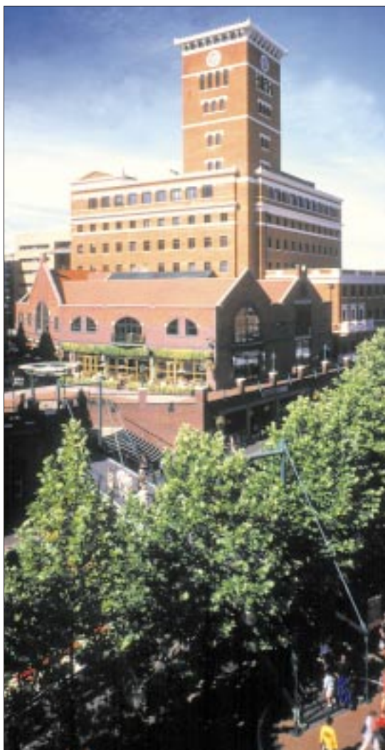
◀ BIRMINGHAM'S BRINDLEYPLACE IS A MAJOR COMMERCIAL MIXED-USE DEVELOPMENT
