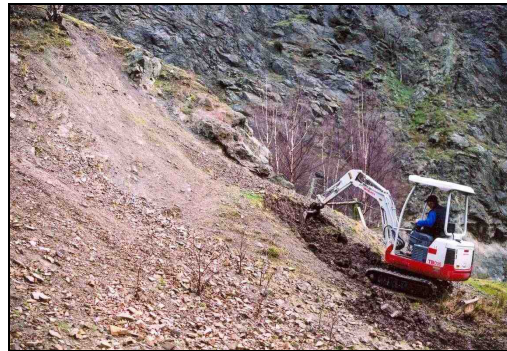
Geoconservation work in the Malvern Hills
