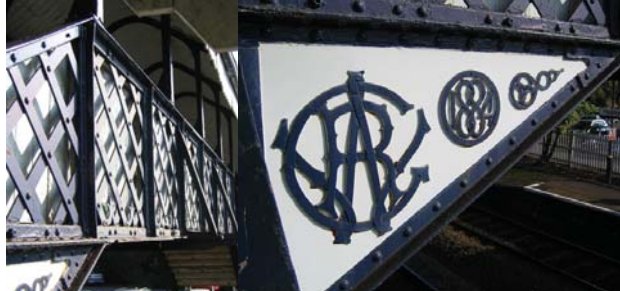
'Hagley Railway Station and Footbridge' Station Drive, Hagley
