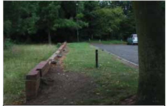
Perimeter wall along Swanslength
